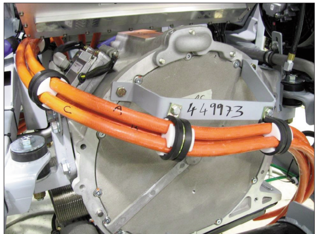
High voltage cables in orange coloured loom
