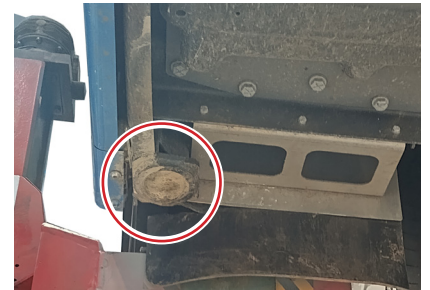
Rear RHS Jacking Point.
